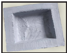
Water ponding test Passed
